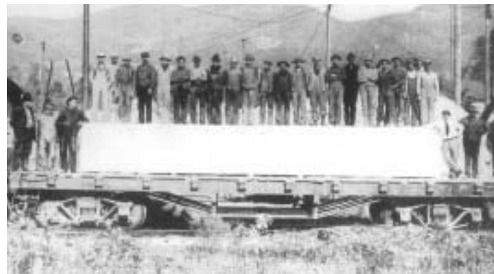
28 men are photographed on the M.D. & G. with one of the 43-ton monoliths bound for the mill after being turned and fluted to serve as one of 13 columns for the D.A.R. building in Washington, D.C.
